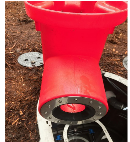
STEP 7: Pull back of the filter carriage to clear the metal wash assembly then lift the filter carriage carriage out.
