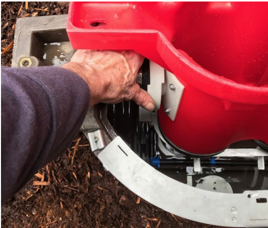
STEP 6: Rotate the fastening nut left or right 90 degrees to free the collar from the filter carriage and pull back on the accordian tube.
